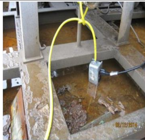
1) Illegal "homemade" extension cord/unmounted receptacle 2) Plug set/receptacle in water.
