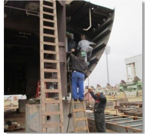
1) Exposed to a fall >5' w/o fall protection. 2) Supervisor deployed workers to job location that did not have adequate fall protection.
