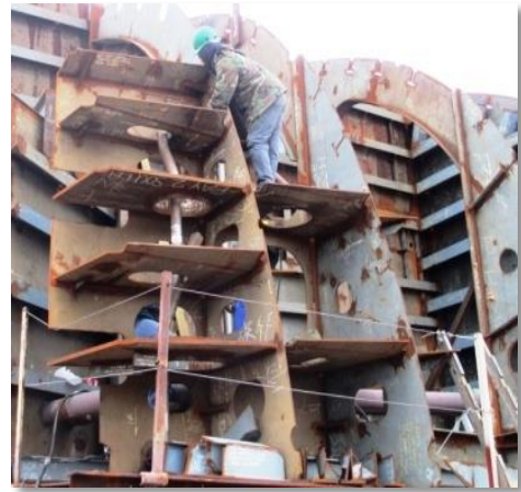
Exposed to fall >5' w/o fall protection.
