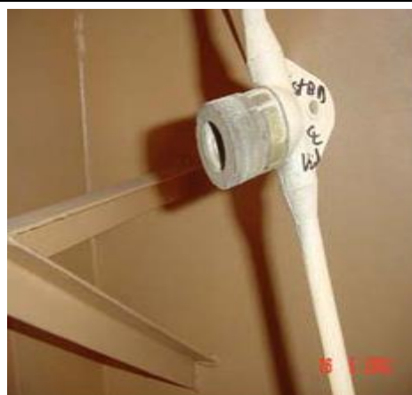
The bulb and globe are missing creating a shock or electrocution hazard.
