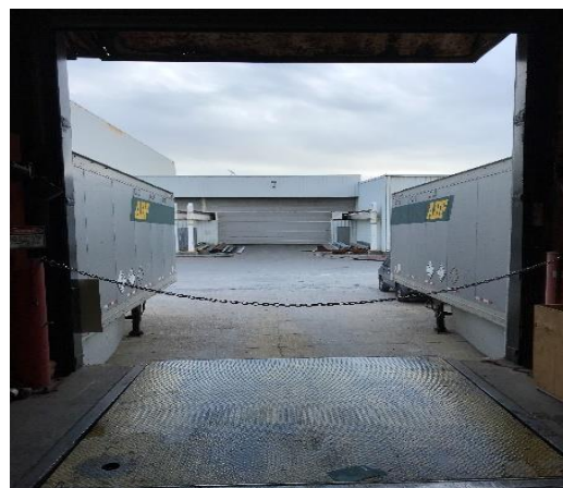
Safety guard chains must be installed whenever doors are open and tractor-trailer is not backed up to the dock.
