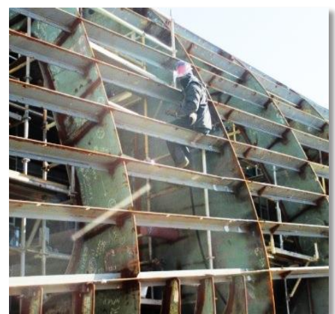
Working >5' without fall protection.
