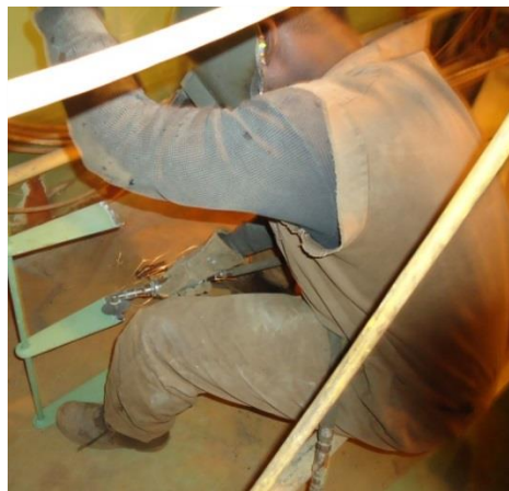
Grinding without a guard on grinder.
