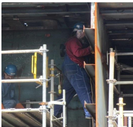
Exposed to a fall >5' without using fall protection.
