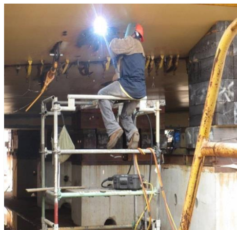
1) Sitting on guardrail. 2) Exposed to a fall >5' w/o fall protection or PFAS
