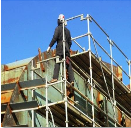
Standing on guardrail of scaffold.
