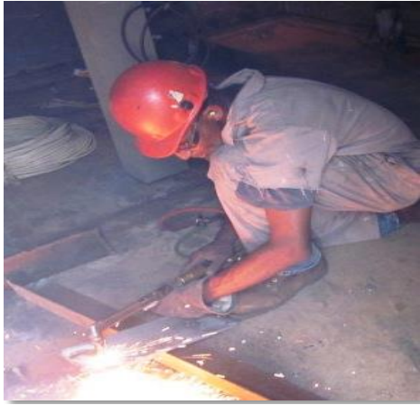
1) Hot work without sleeves. 2) Using cutting torch without burning goggles. 3) Hot work with only one glove.
