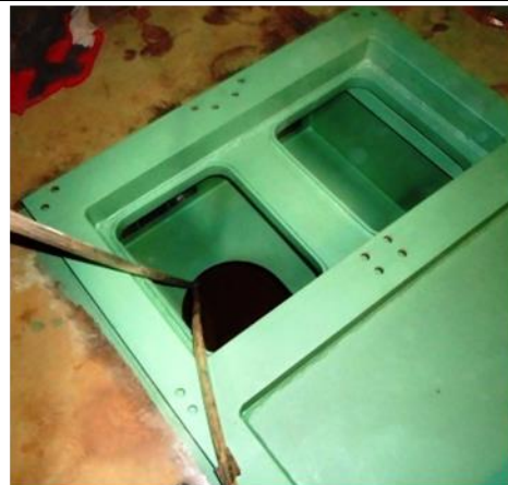
Uncovered/unguarded open hole on deck.
