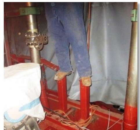
Not using a proper walk/work surface to conduct work.
