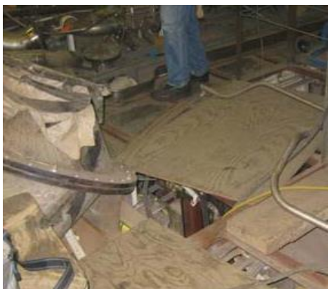
The deck plate has not been replaced and has left an opening in the deck.
