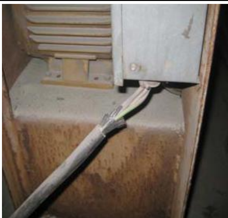
The strain relief has failed and allowed the cable to be pulled out exposing the wires inside of the cable.
