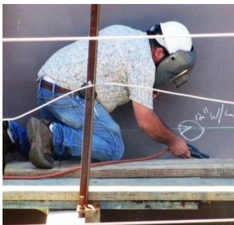
1) Supervisor, working on a scaffold with a damaged guardrail. 2) Conducting hot work w/o gloves. 3) Conducting hot work w/o sleeves. 4) Not wearing hearing protection. 5) Conducting hot work w/o wearing 6" high safety footwear.
