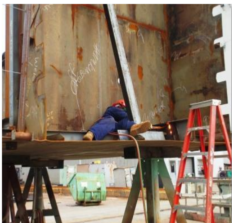
1) Working >5' without fall protection on deck edge. 2) Accessing structure with a stepladder.
