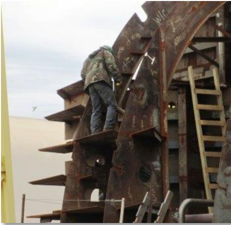
Exposed to fall >5' w/o fall protection.
