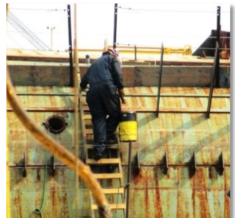
Not maintaining 3-point contact on ladder due to carrying item in hand. Always use a hand line to pull up tools and materials.
