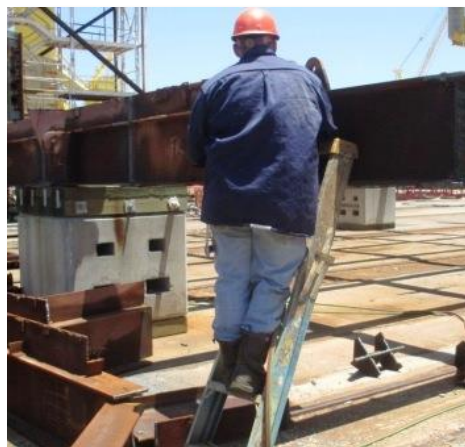
1) Improper use of stepladder. 2) Using torch with pants tucked in boots.
