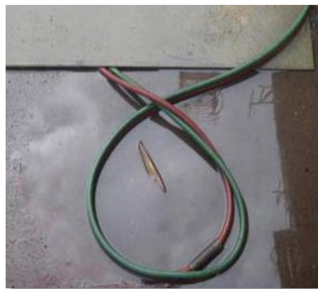
Material has been placed on this torch hose, which can damage it and create a fire or explosion hazard.
