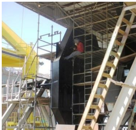
Exposed to fall >5' w/o fall protection.
