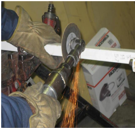
1) Grinding with the guard removed from grinder. 2) Conducting hot work w/o removing combustibles 35' or more.
