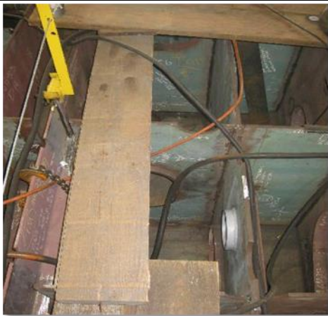
Poor line control. Walkways must be kept clear of lines. Walking on lines will damage them and create other hazards.
