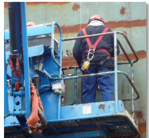
Wearing PFAS improperly while operating aerial lift.
