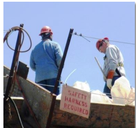
1) Not complying with sign stating, "Safety harnesses required". 2) Working exposed to a fall >5' with openings in guardrail.
